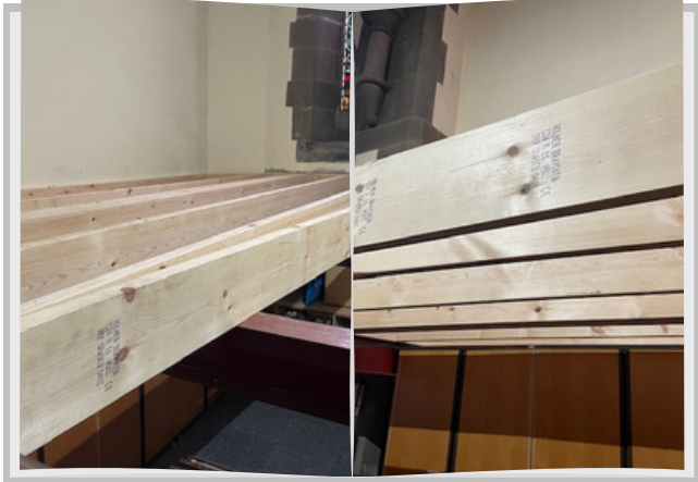
flooring for the new studios
